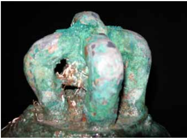
Fig. 59. Detail of the two single and two double canon rings on the top of the ship's bell.
